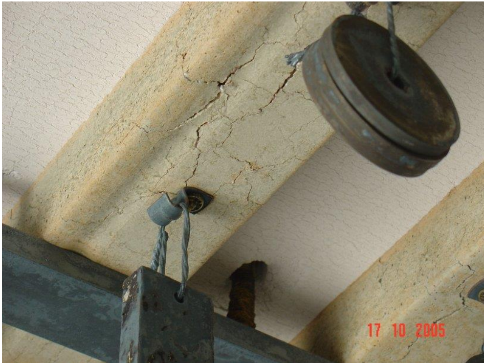
Foto 7: . Detail beugel in beton na de test.
