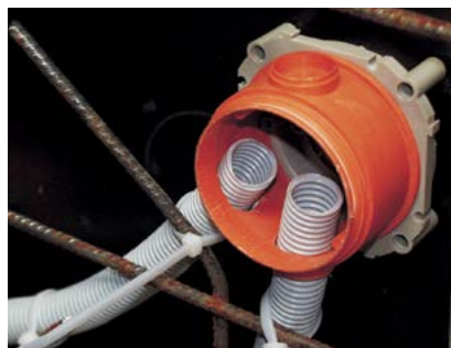
Flexible pipes installed into KBT body.
